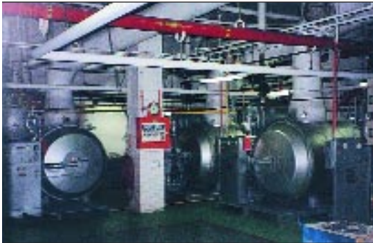
FIGURE 2. 200 bhp recirculating coil-type steam generators in basement of Fourth & Vine Tower, Cincinnati, Ohio.
