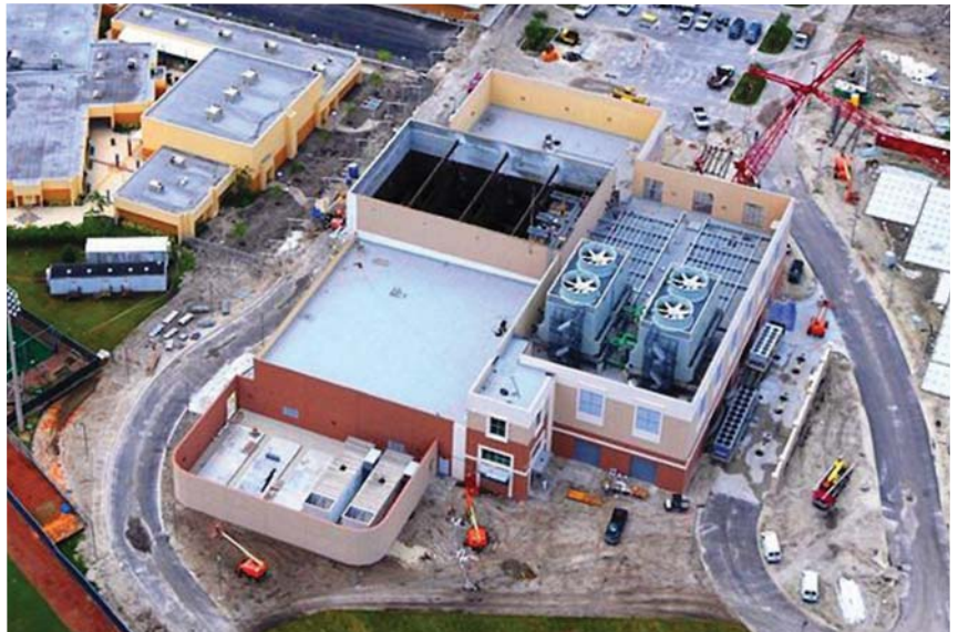
The Nova Southeastern University central energy plant.
