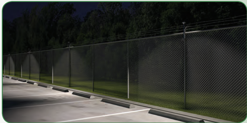
Typical perimeter lighting application.
