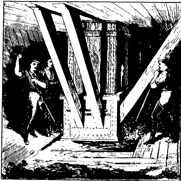
Men at work inside during the caisson's descent, Brooklyn Bridge.
