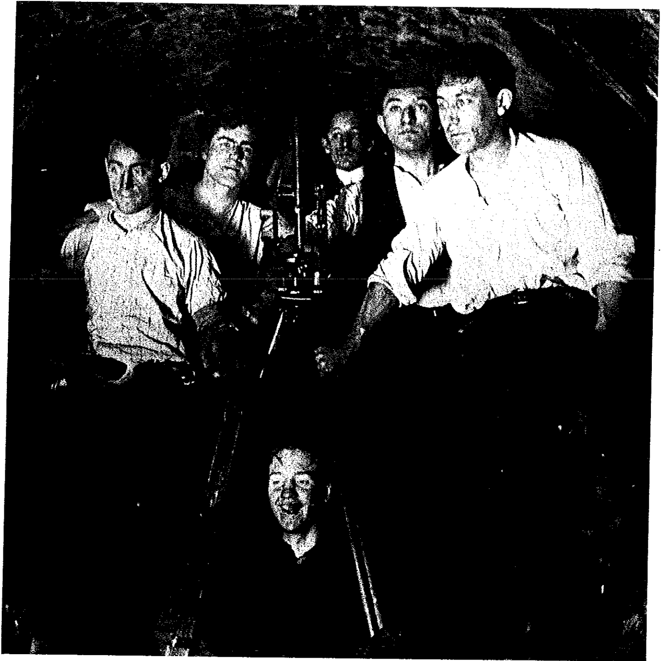
Subway construction workers in tunnel (photograph undated).
