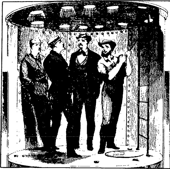
Men at work inside during the caisson's descent, Brooklyn Bridge.
