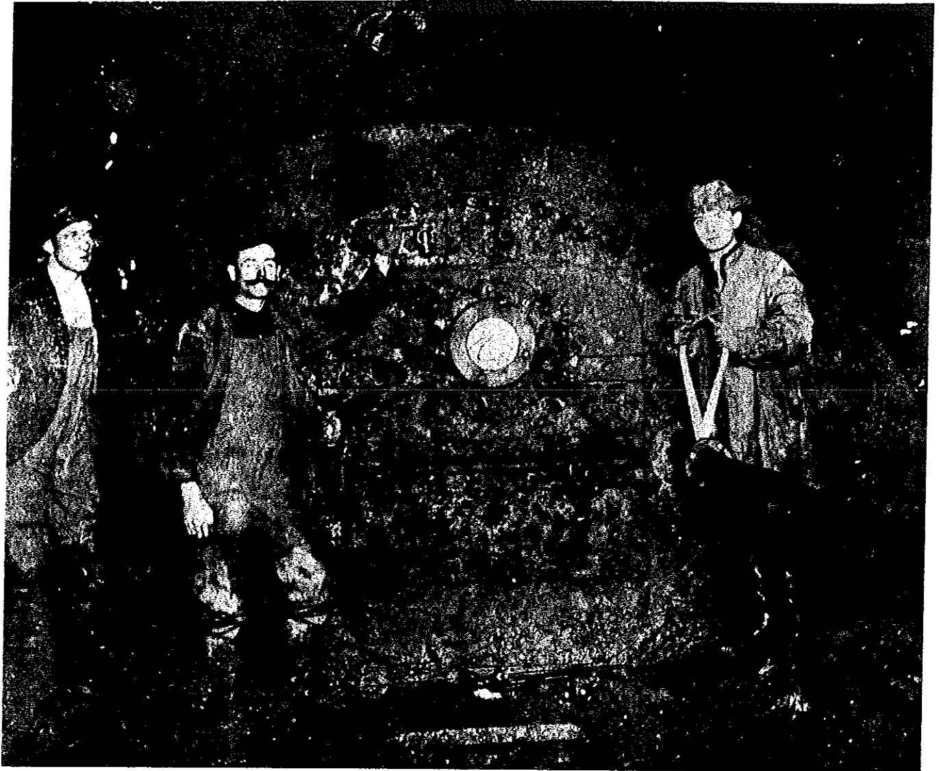
The McAdoo Tunnel — air lock.
