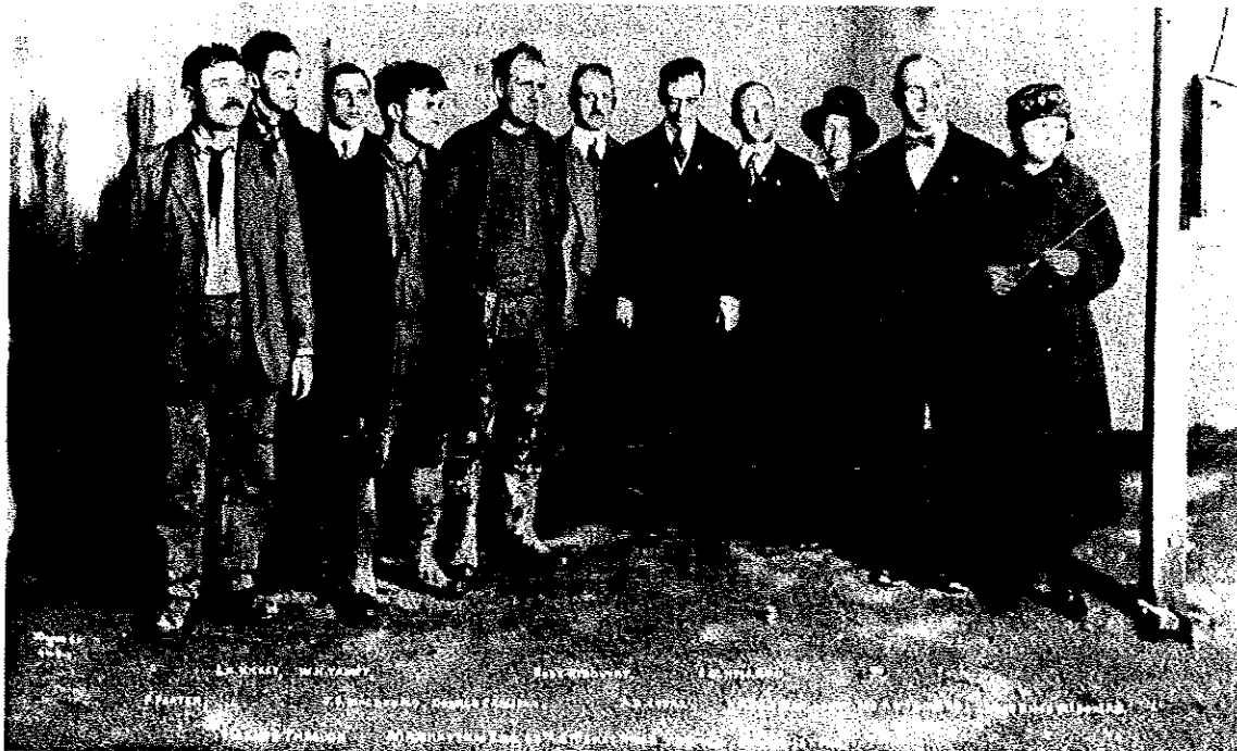
Subway under East River — "Holing Through"; October 13, 1918.
