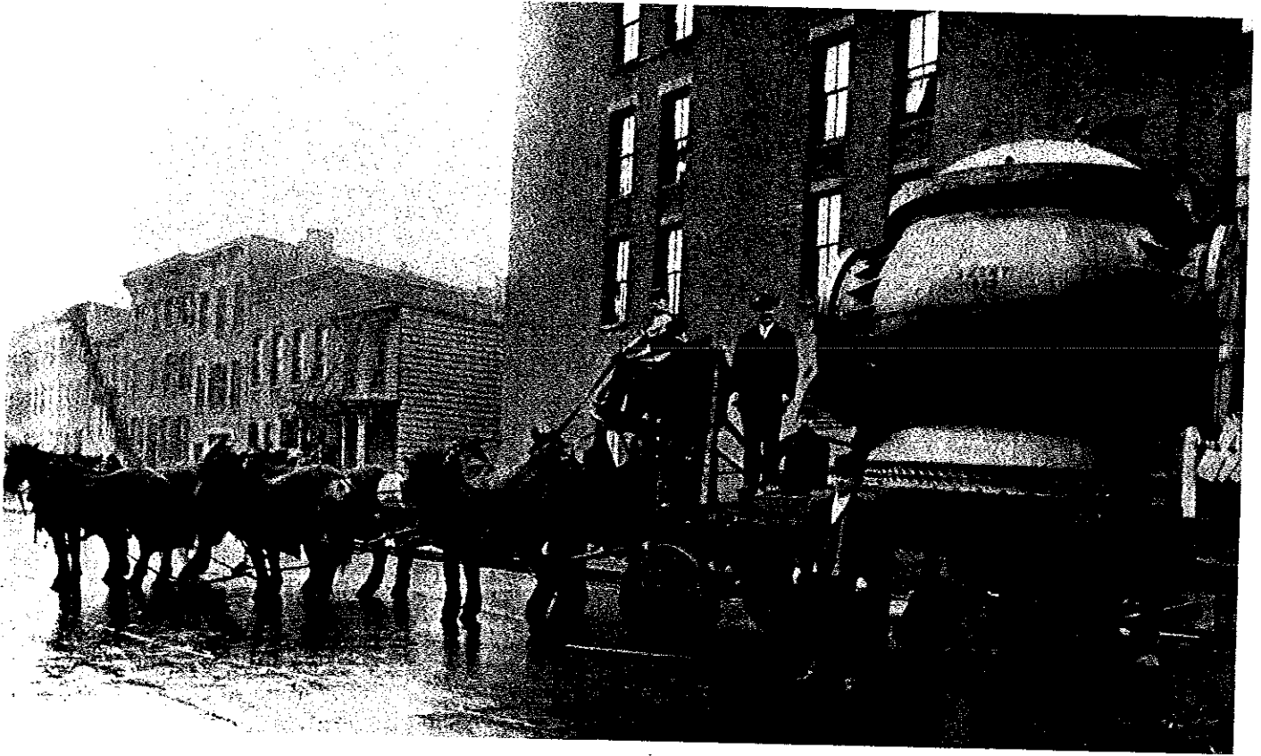
Catskill Aqueduct — City tunnel. 72" x 48" Bronze shaft cap to which city water mains are connected.
