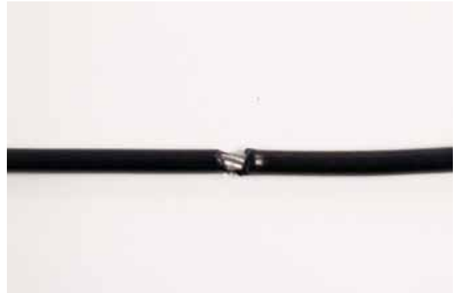
A CRACK IN THE CABLE COVER
